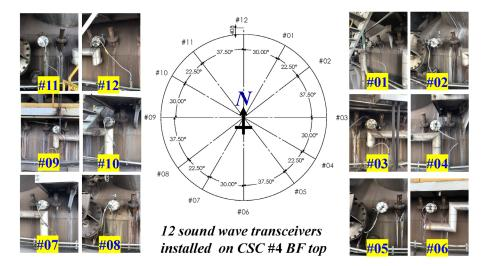
Fig.12. Arrangement of 12 sound wave transceivers on CSC #4 BF.
